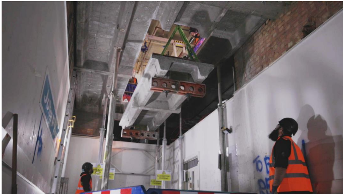
Figure 19: Extraction of in-situ slab at Euston Tower
